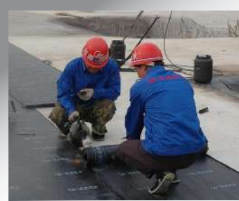
Modified Bitumen Membrane
