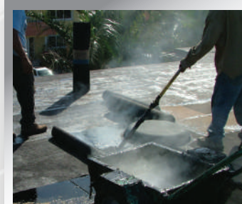
Hot Mopped Roofs
