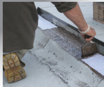
Liquid Applied Polyurethane Waterproofing
